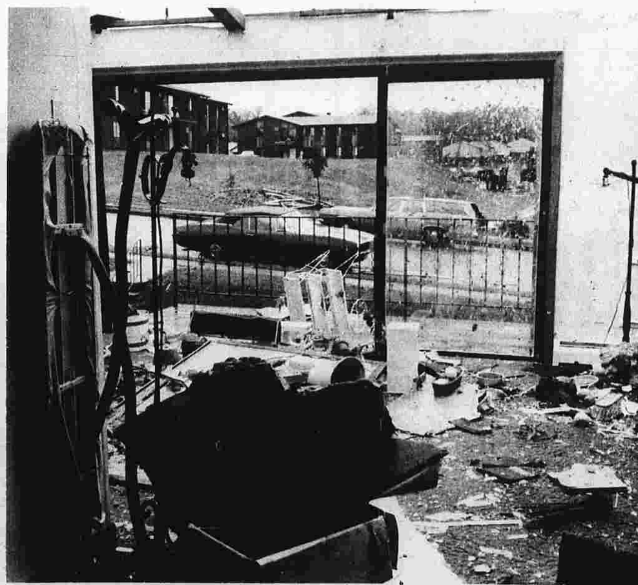
These are views of the tornado that swept through the North End of Manchester and on into neighboring Talcottville, Vernon and Tolland on Sept. 5, 1973. A doll lies among the rubble near the apartments on Rachel Rd., parts of roofs that were blown off. Below is a scene from inside one of the apartments.
