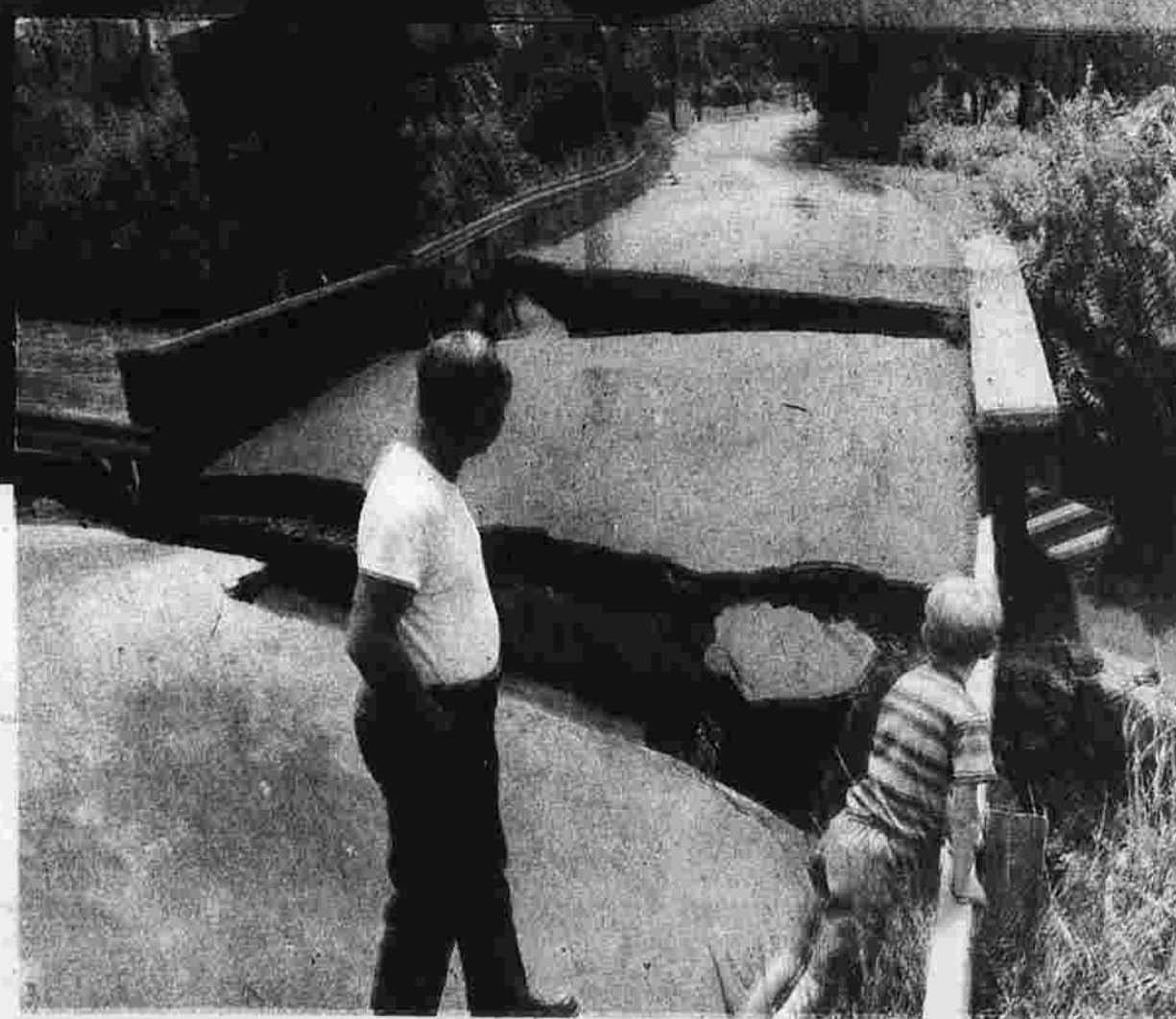
June Washout of the Olcott St. Bridge
