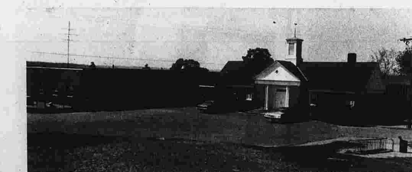
The Andover Elementary School, School Rd. The original building was constructed in 1948.
