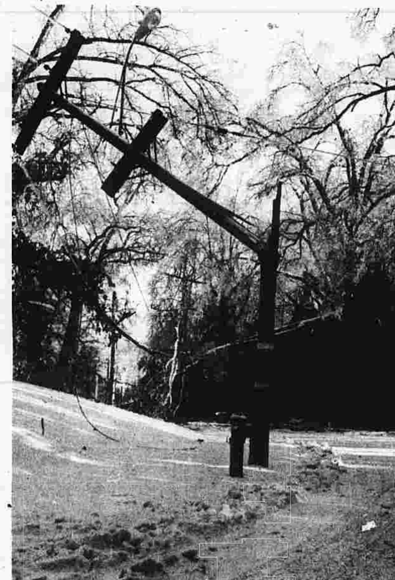
Utility poles were snapped under weight of ice.
